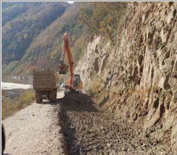
Km 0+230 ~ Km 0+380(RHS) ; Excavation for Capping Layer
