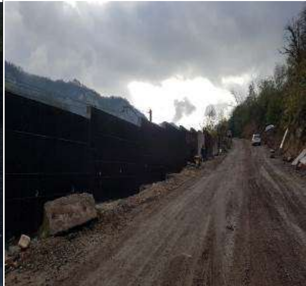
Km6+485 ~ Km6+600(LHS) ; Bituminous Coating for RC Wall
