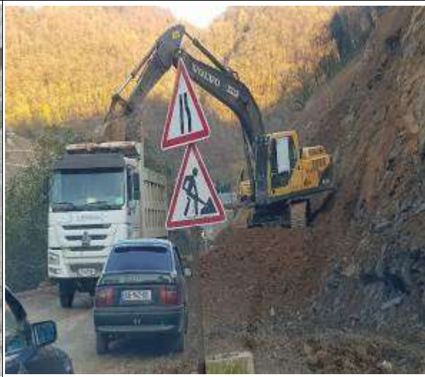
Km 2+495 ~ km2+515(RHS) ; Excavation of Slope
