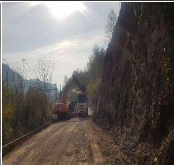
Km 6+440 ~ Km 6+460(RHS); Excavation of Slope
