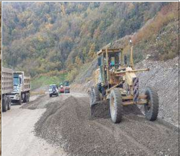
Km0+400 ~ Km0+780(RHS) ; Construction of Granular Bas
