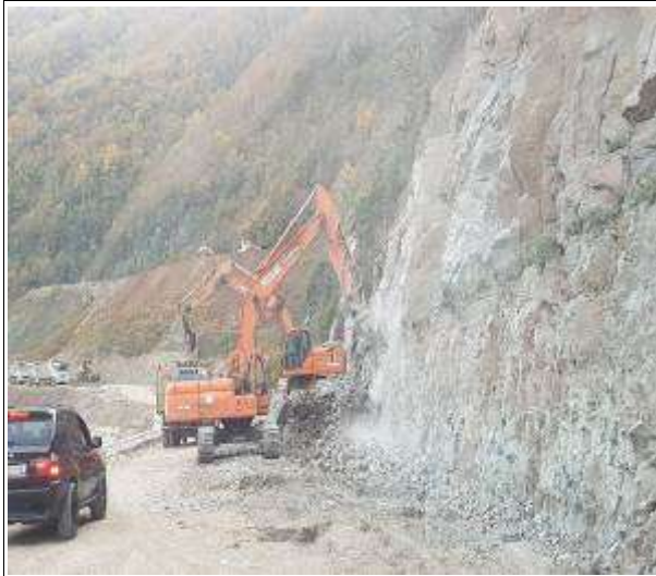
Km 0+360 ~ km 0+390(RHS); Excavation of Slope
