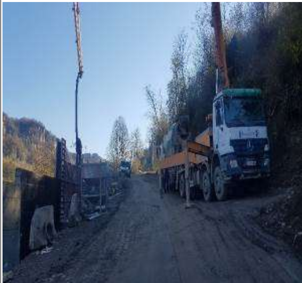
Km6+585 ~ Km6+600(LHS) ; Concrete for RC Wall
