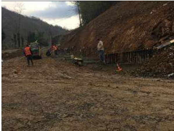
Spoil stockpiles alongside the road
