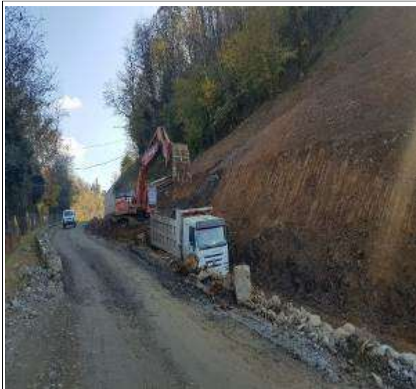
Km 2+580 ~ Km 2+700(RHS); Excavation of Slope
